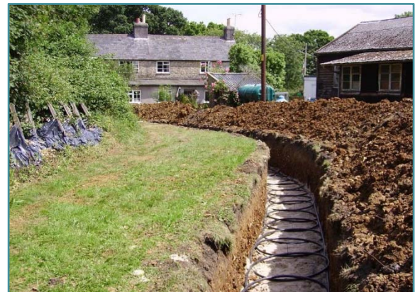
Figure 5 – Shallow horizontal ground loops
